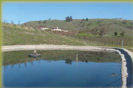
Water reclamation storage.
