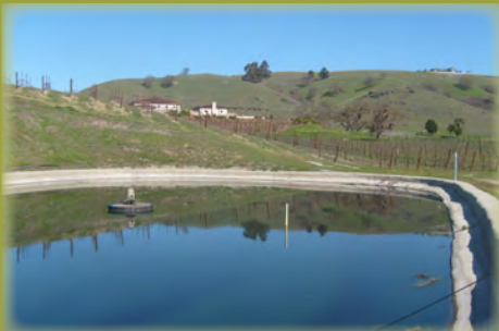
Water reclamation storage.
